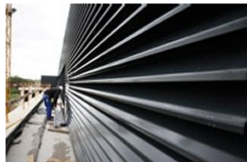
No visible joints between Louvre Panels is one of the main features of Continuous Louvre Systems
